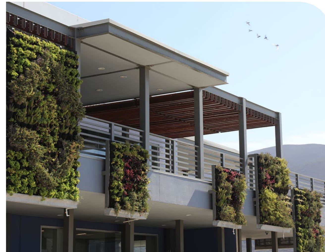
Ensenada, Mexico MODCO facility
