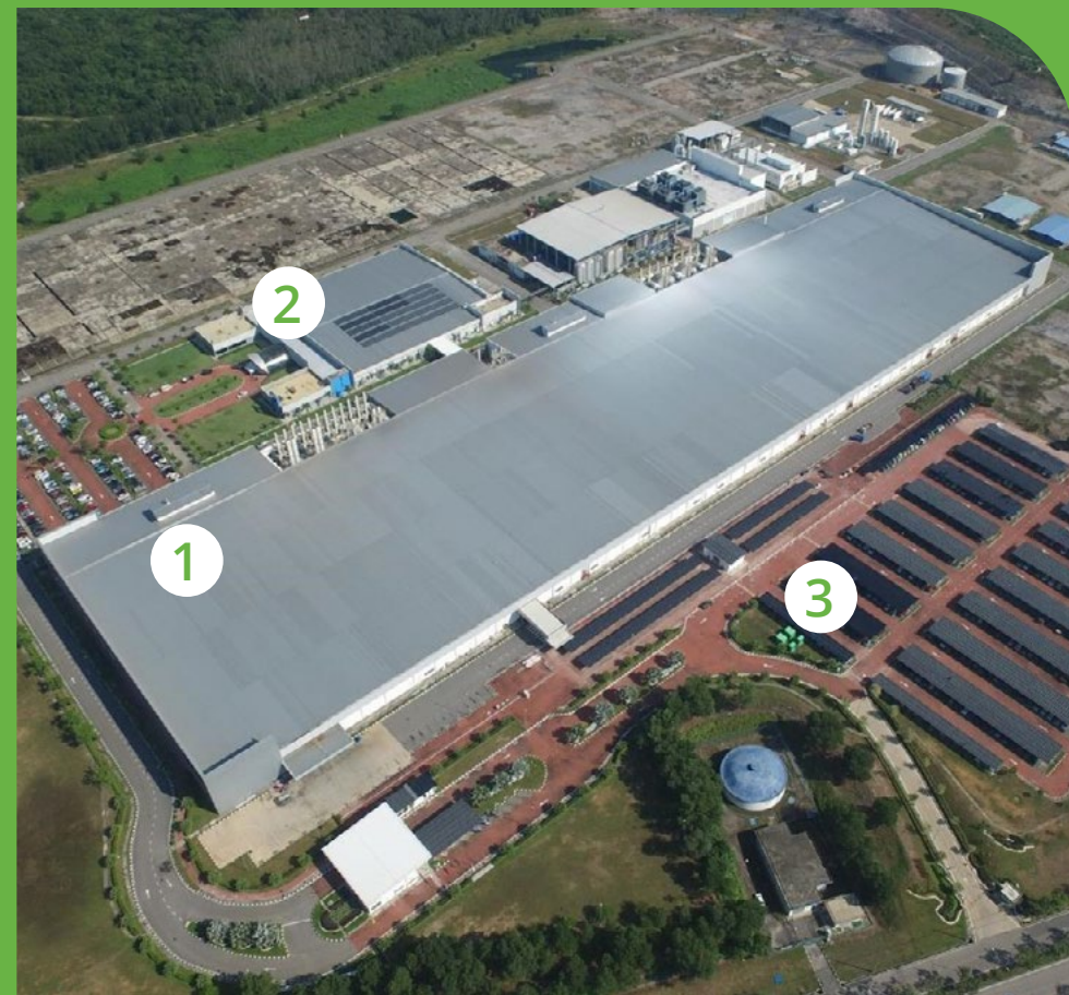
1. Future planned – FAB rooftop
