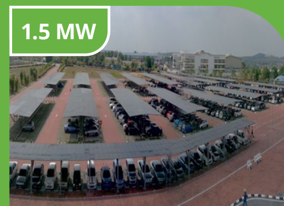
3. Covered carpark and motorcycle area
