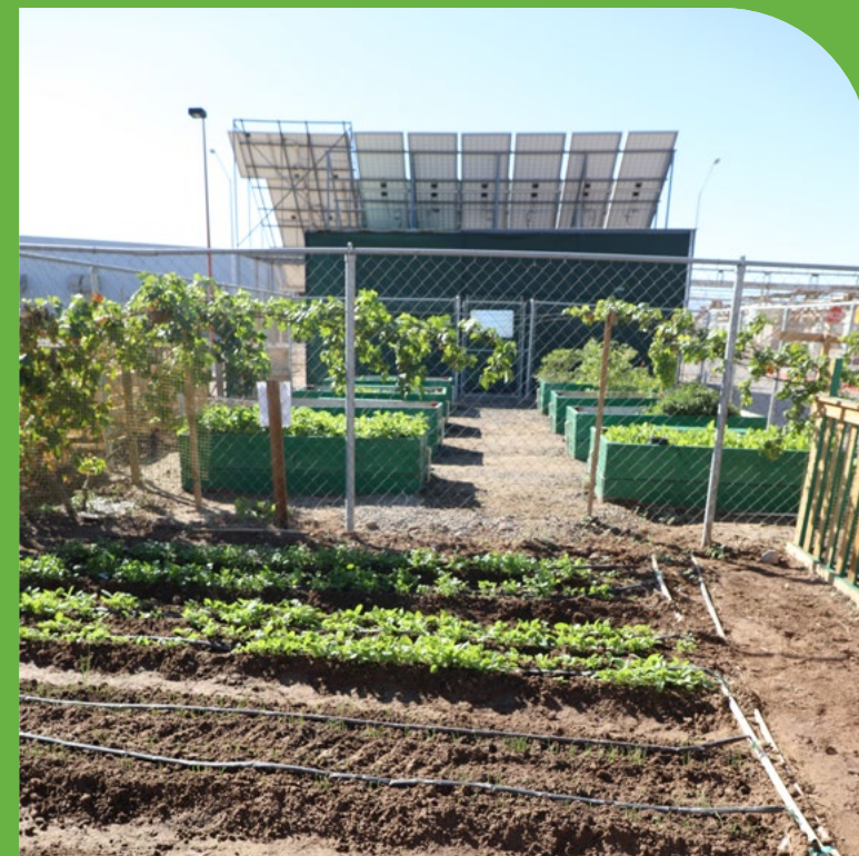
Solar panels installed atop our organic garden
