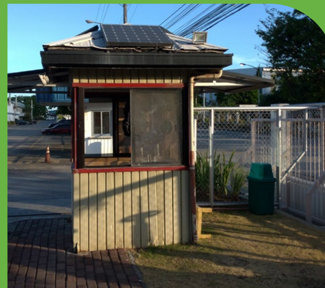
Installation of Solar Panel at the Security Post
