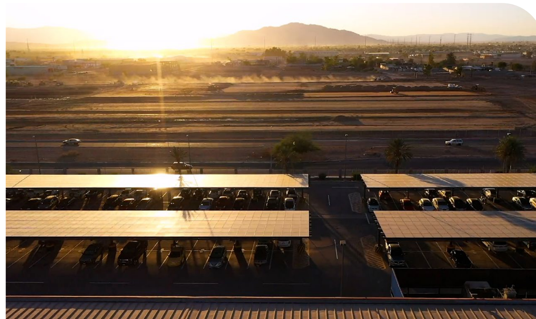
Carport solar in Mexicali, Mexico facility
